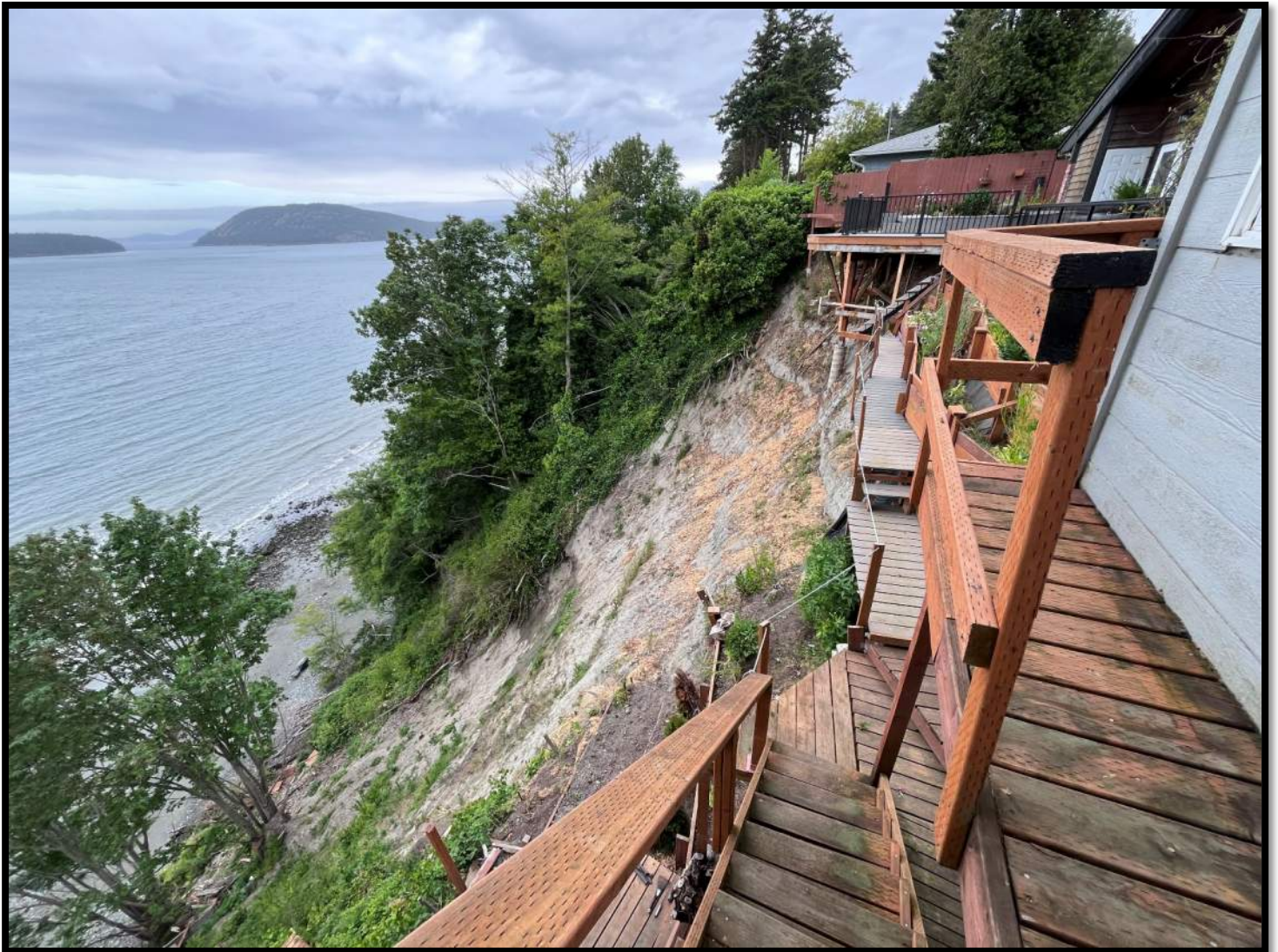
Photo 1: Existing conditions at the bluff slope face showing the landslide footprint. Facing N on May 29, 2026.
