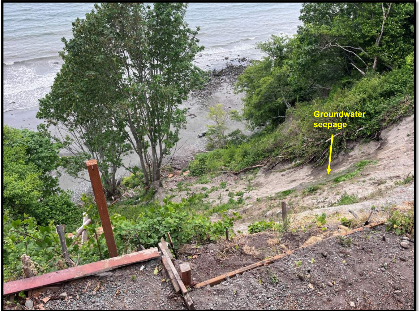
Photo 2: Existing conditions looking down the slope toward the beach area. Note seepage in upper central slope. Facing NW on May 29, 2026.
